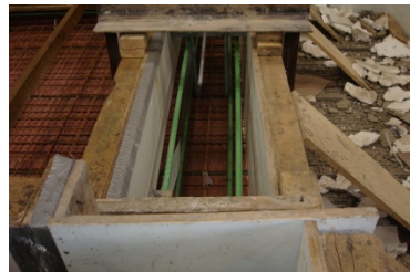
Figure 14 – Insulation Being Installed in the Mold
