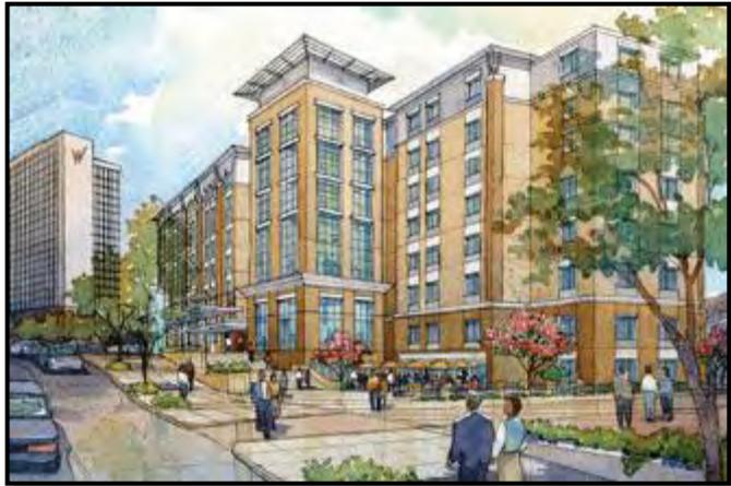
The exterior of the hotel is mainly brick and cast-stone veneer, architectural decisions made to resemble the bordering CONSOL Energy Center. A lighter color brick is used from the 2<sup>nd</sup>-Roof Floor levels, with the addition of a cast-stone band at the second and seventh floor level. The darker color brick is used from the second floor level and below, as well as vertical strips to separate window pairings and to accent building corners.
