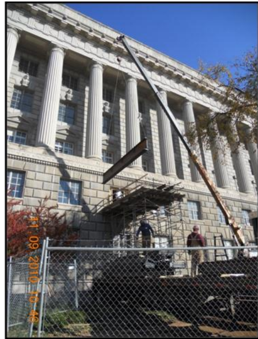
Figure 21: Delivery trucks back into an area near the building's opened corridor where a small crane is used to hoist the steel members onto rollers
