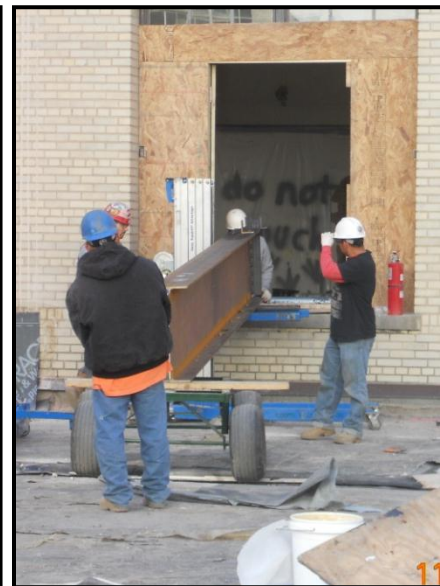
Figure 22: Once set, steel members are rolled through the building into the EEE courtyard. Workers use rollers and hand jacks to place the member in its appropriate place on top of the existing structure
