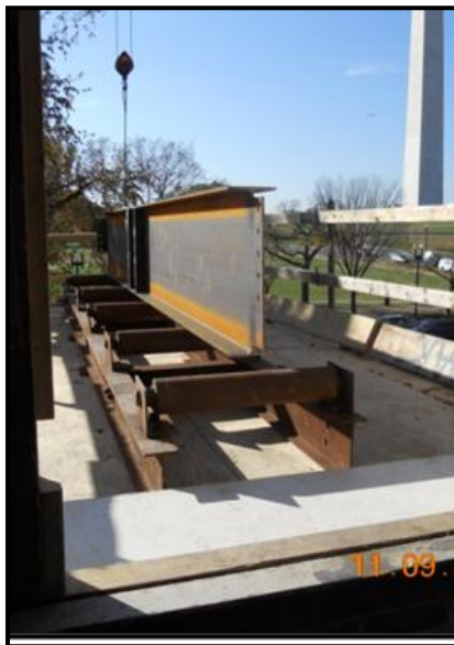
Figure 22: Once set, steel members are rolled through the building into the EEE courtyard. Workers use rollers and hand jacks to place the member in its appropriate place on top of the existing structure
