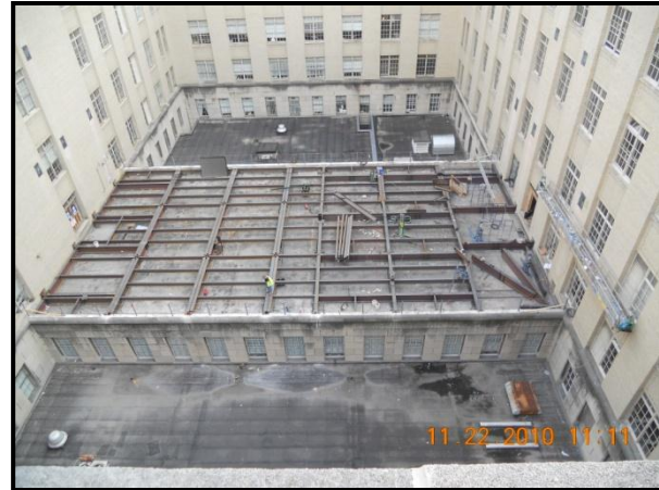
Figure 23: Because the small crane can be used without occupying the adjacent roadway, steel erection can take place throughout the week
