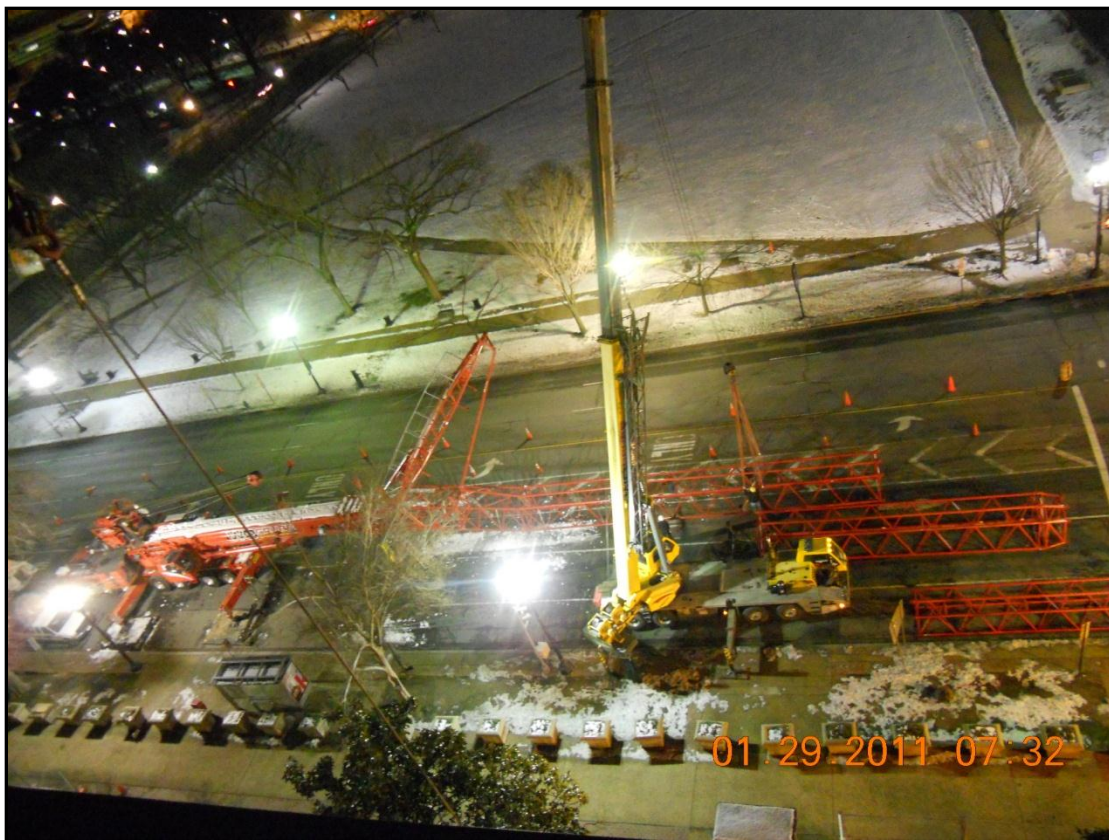
Figure 14: Erecting the cranes jib. A smaller crane was used to attach the components along the southern end of the staging area
