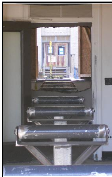
Figure 22: Once set, steel members are rolled through the building into the EEE courtyard. Workers use rollers and hand jacks to place the member in its appropriate place on top of the existing structure
