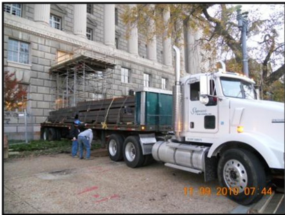
Figure 21: Delivery trucks back into an area near the building's opened corridor where a small crane is used to hoist the steel members onto rollers
