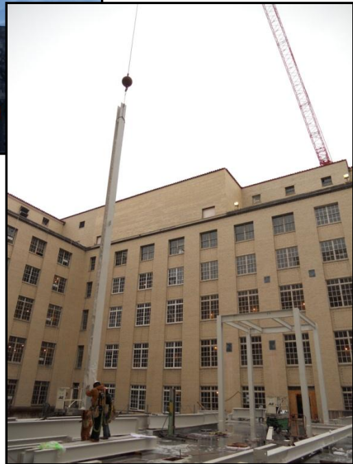
Figure 15: Steel column being set within the courtyard of the building for the EEE
