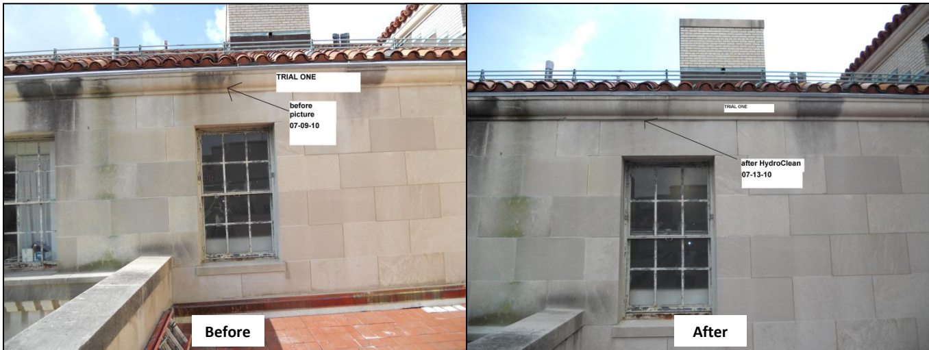
Figure 8: Mock-Up Photos from HydroClean HT Application
