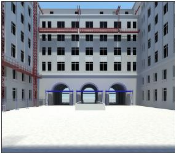
Figure 2: Overhead protection will be erected throughout all entrances corresponding to the parking courtyards. A total of 5 occupant vehicles will be parking in the center of courtyard 2 during exterior restoration work.
