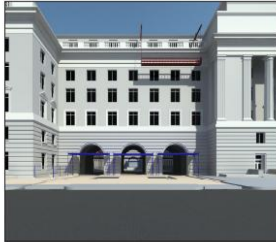
Figure 2: Overhead protection will be erected throughout all entrances corresponding to the parking courtyards. A total of 5 occupant vehicles will be parking in the center of courtyard 2 during exterior restoration work.
