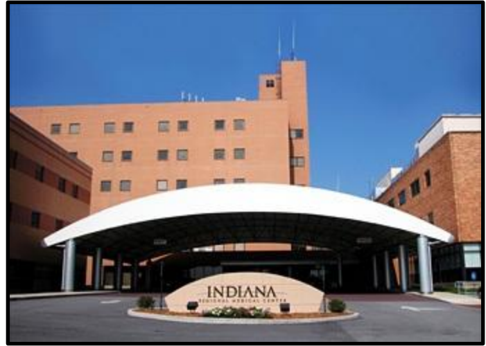
Figure 1 – Current Entrance to IRMC
