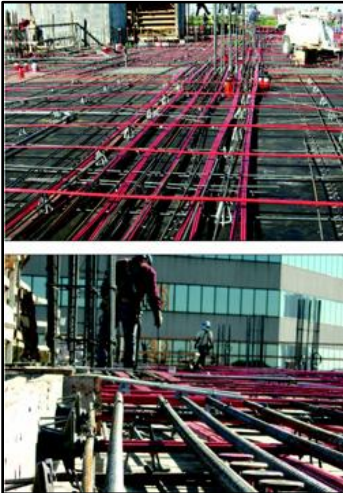
Figure 16 – Example of a Post-Tensioned System
