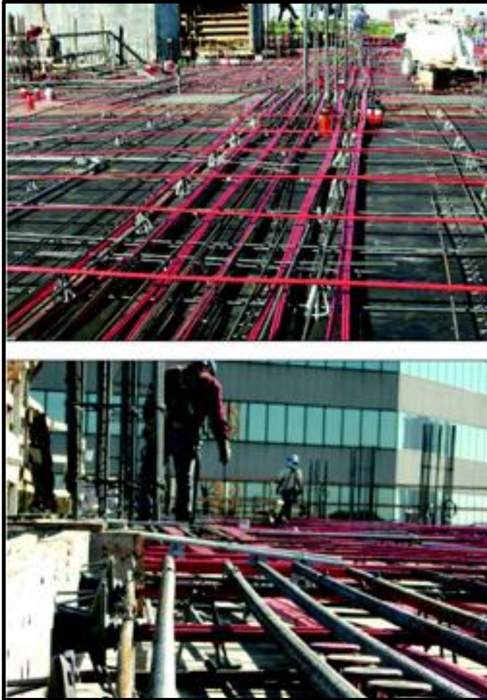
Figure 27 – Example of a Post-Tensioned System
