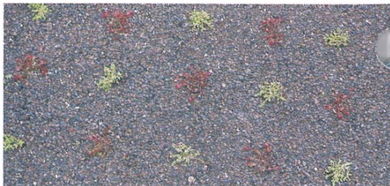
Figure 25: Conventional Green Roof System Day 1
