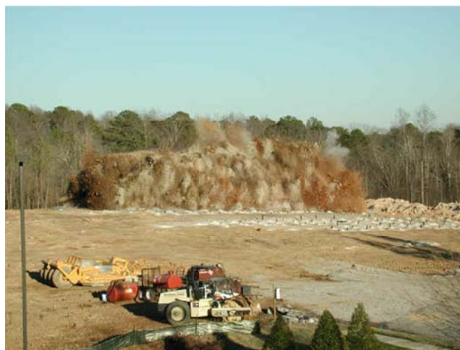
Figure 4: Mass Blasting
