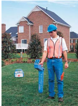
Figure 1: Utility Line Locator
