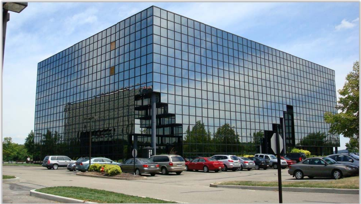
Figure 1- Exterior Picture of the Curtain Wall
