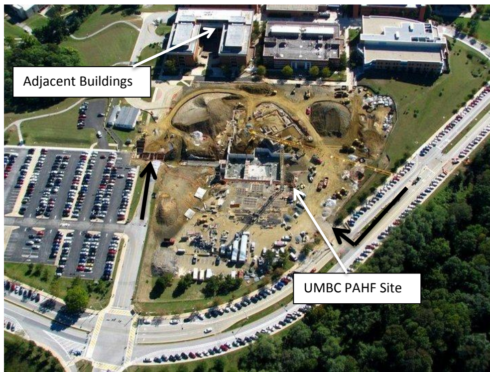
Figure 2: Aerial View of UMBC PAHF Construction Site
