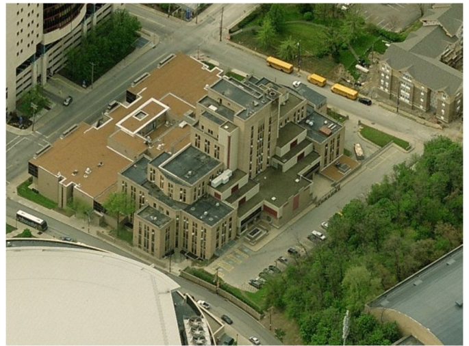
Figure 1-Existing Salk Hall Laboratory
