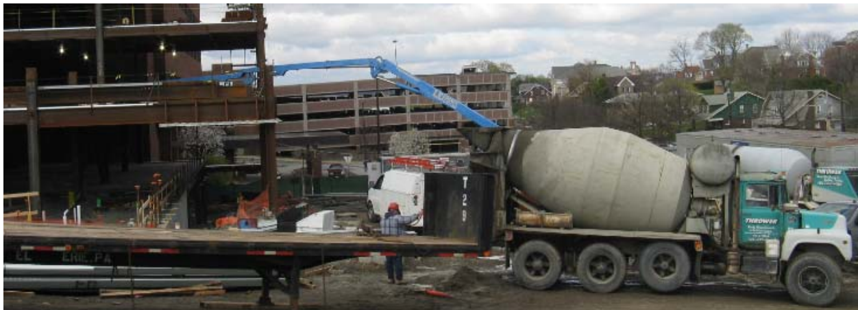
Concrete Slabs being Pumped
