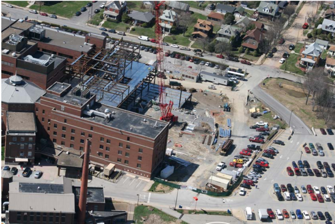
Image from Northwest: Manitowoc setting steel
