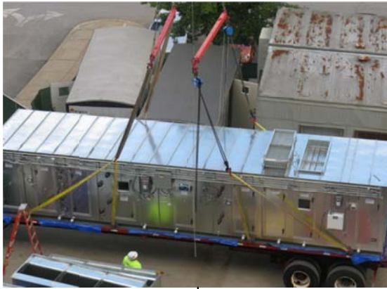
AHU Being Hoisted
