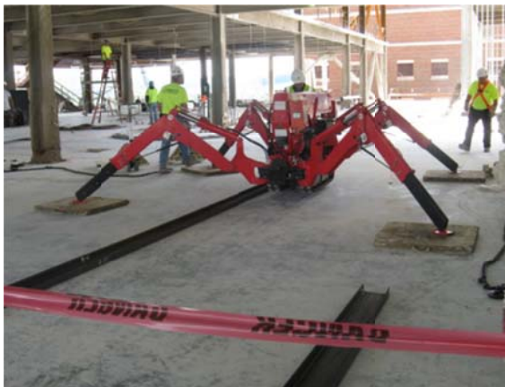
Spider crane set to move Unit
