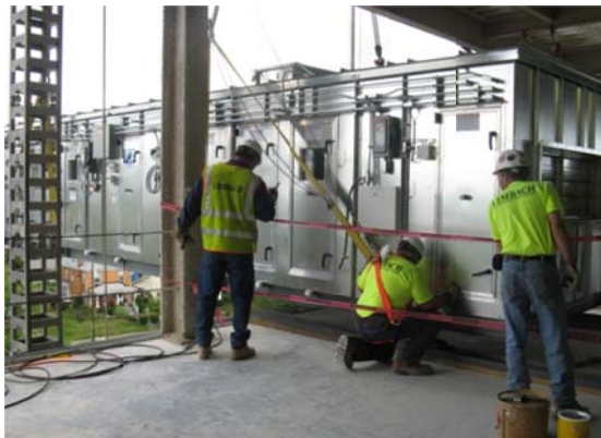
AHU set onto 5 th floor
