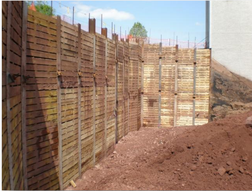
Figure 10. Soldier Piles and Lagging as used in an Earth Restraint Application. Compliments Moretrench.com
