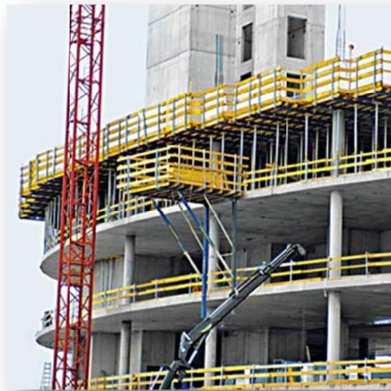
Figure 2. Dokamatic Formwork System. Courtesy Doka Website.
