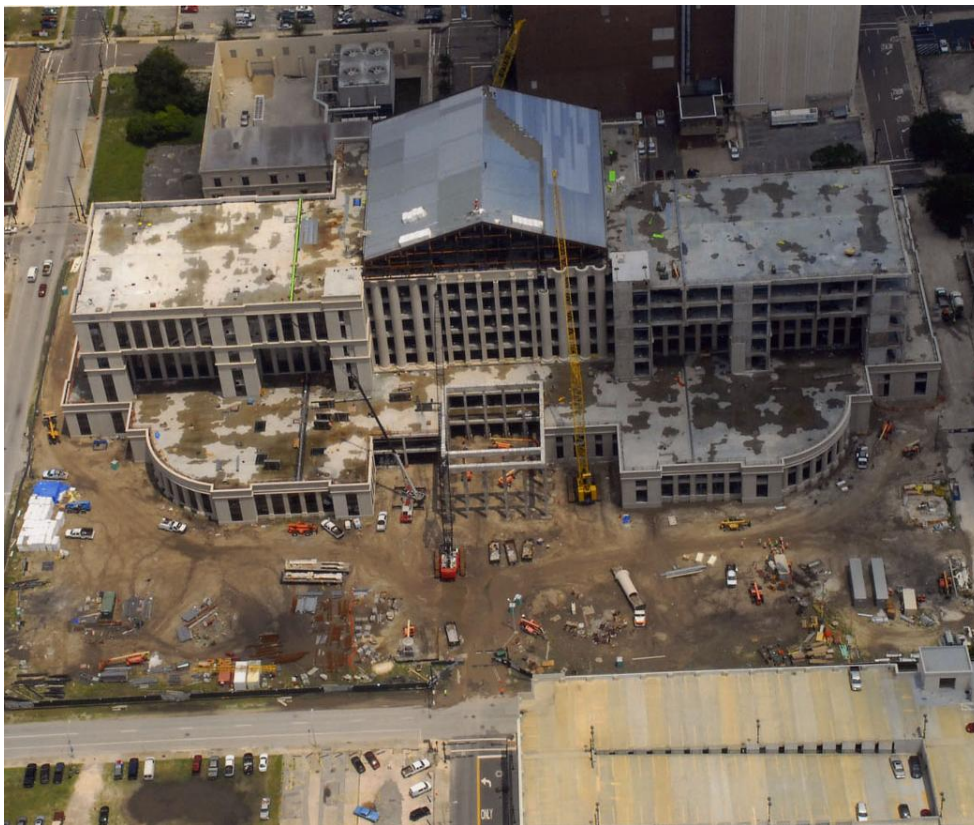
Figure 5. Aerial view of crane locations during s lift.
