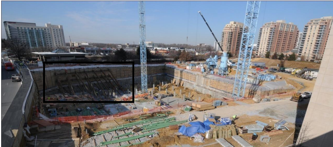
Figure 13: RAKER SYSTEM ON PROJECT
