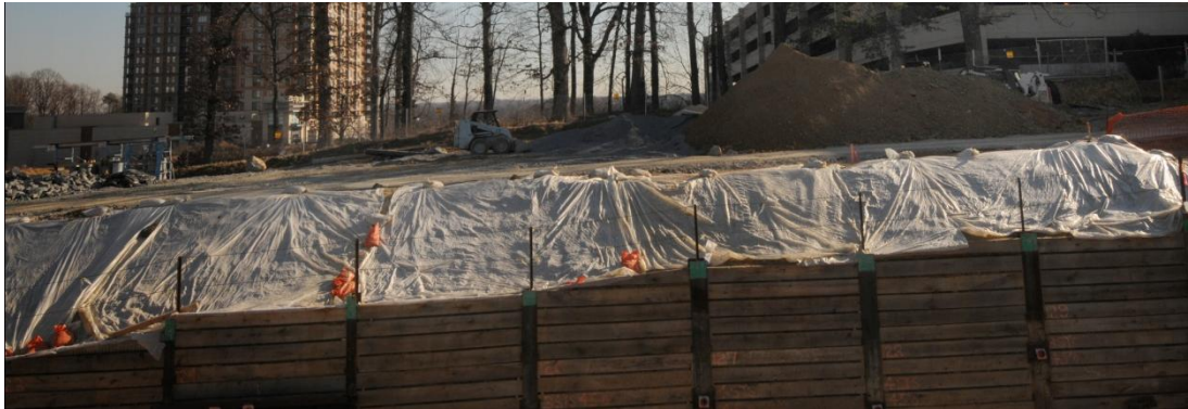
Figure 11: WOOD LAGGING AND SOLDIER PILES
