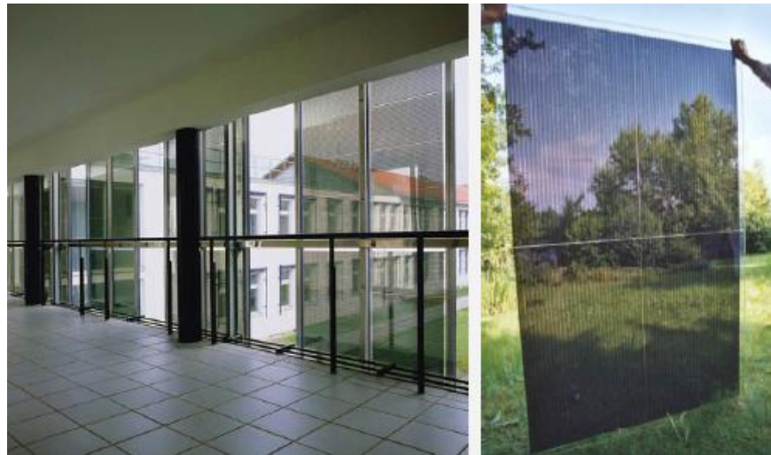
Figure 20: TRANSPARENT PV GLASS CENTENNIAL SOLAR
