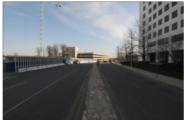
Figure 33: LOOKING EAST (COVERED WALKWAY)
