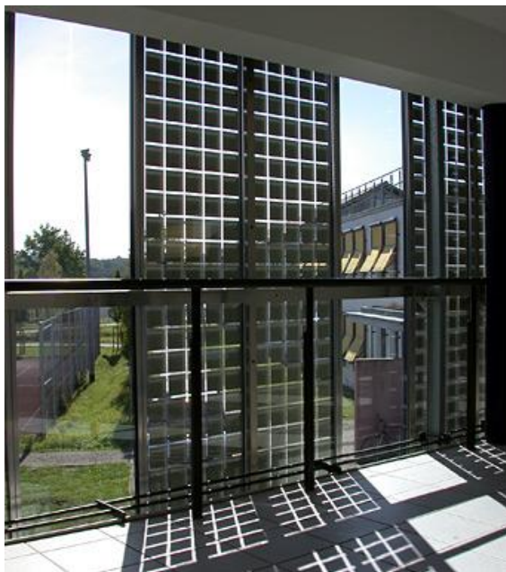
Figure 18: SEMI-TRANSPARENT PV GLASS UNIVERSITY OF SOUTHAMPTON
