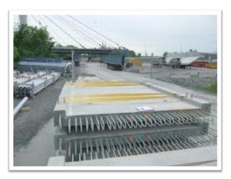
**Figure 4 - Prefabricated Floor Panels**
