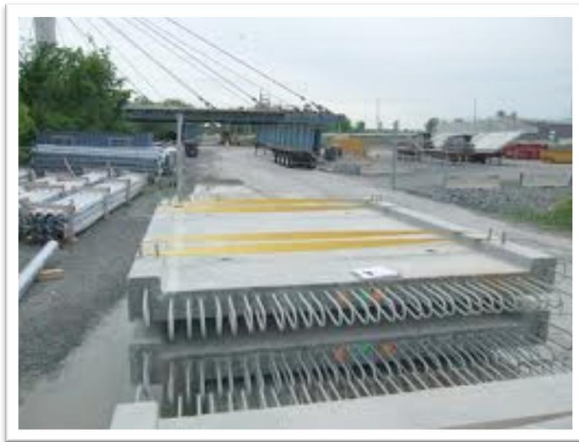
Figure 4 - Prefabricated Floor Panels
