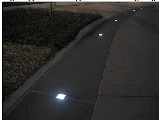
Figure 45: Recessed Ground Lighting
