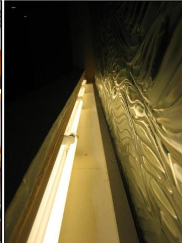
Figure 14: Fluorescent Cove Detail
