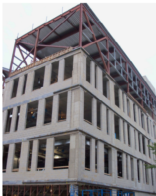
Figure 4: Northern Facing Exterior
