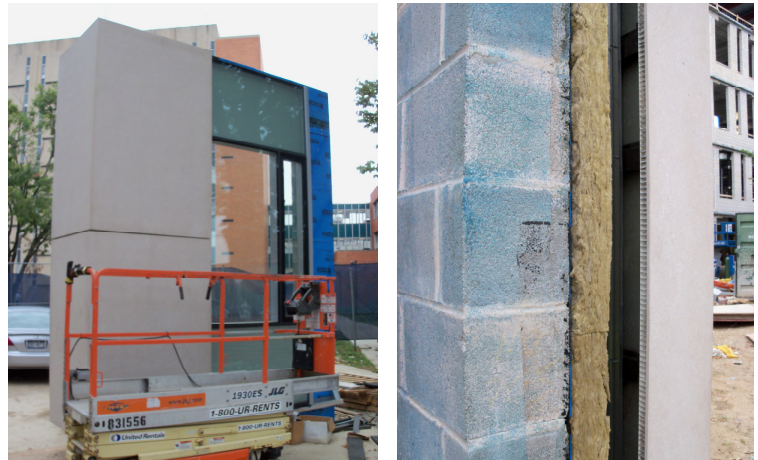
Figure 9: On-site Mock-up of the Exterior Wall
