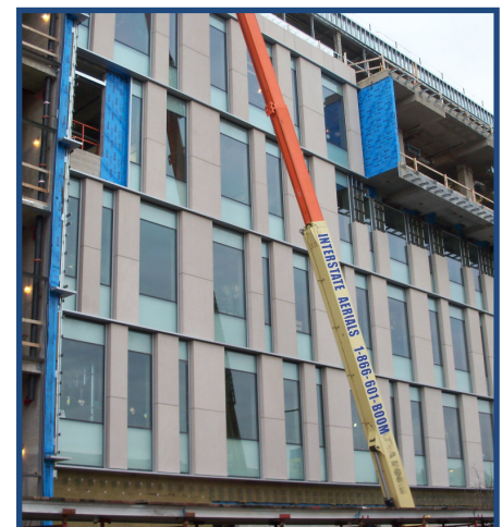
Figure 12: Completed Portion of Exterior Façade
