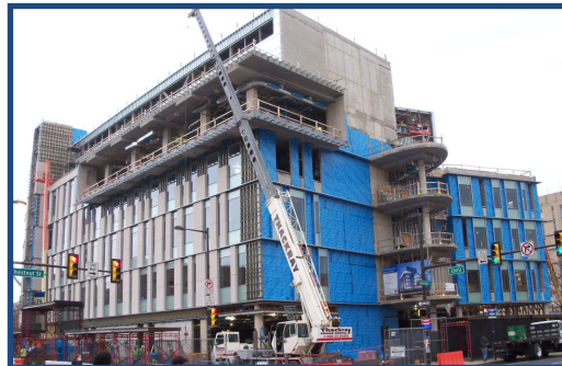
Figure 10: South-West Corner of the Building
