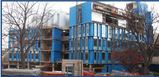
Figure 8: North-East Corner of the Building
