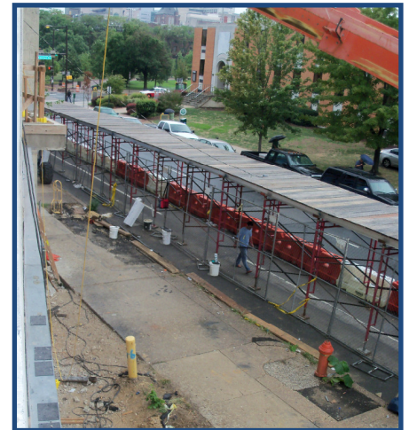
Figure 11: Overhead Protection
