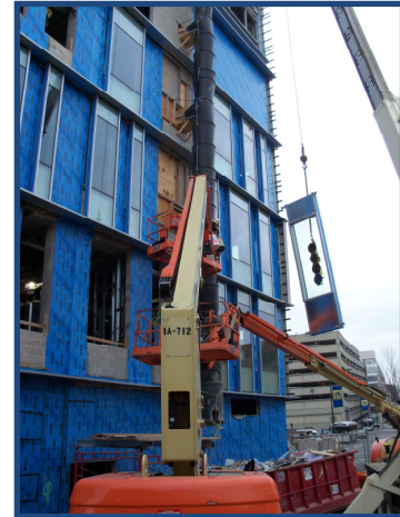
Figure 9: Window Installation
