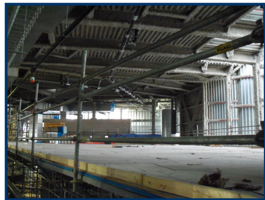
Figure 5: “Dance Floor” Supported by Scaffolding
