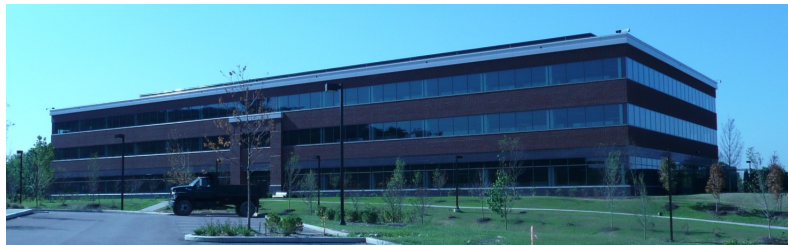
Figure 2: Shows the additional aluminum fascia along the top of the building and a small accent strip in the middle above the entrance.
