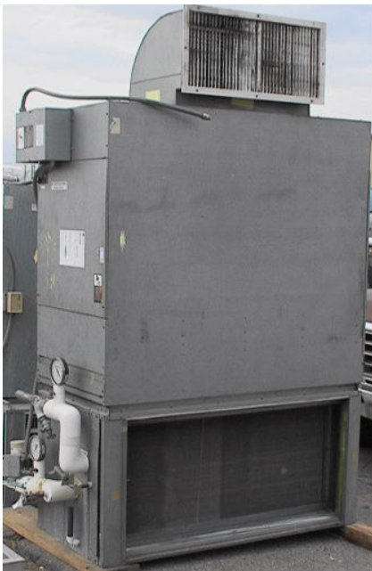
Figure 4: Shows a picture of the Trane Air Handler that was substituted on the project to save cost.
