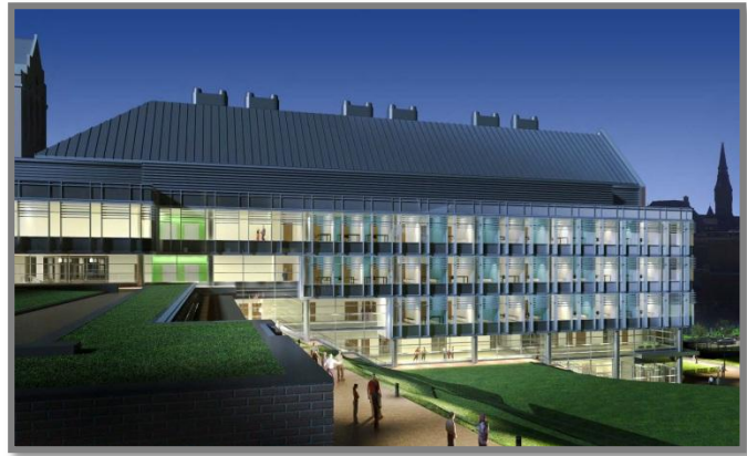
FIGURE 4: NEW SCIENCE CENTER WEST FAÇADE – COURTESY OF PAYETTE
