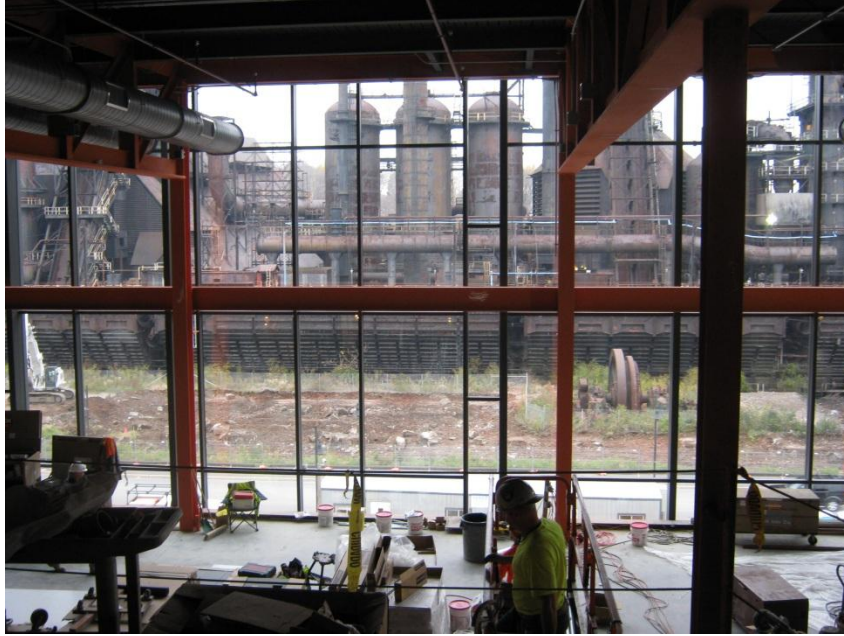
Figure 21- Picture from the Suites looking out to the Blast Furnaces and down onto pit area
