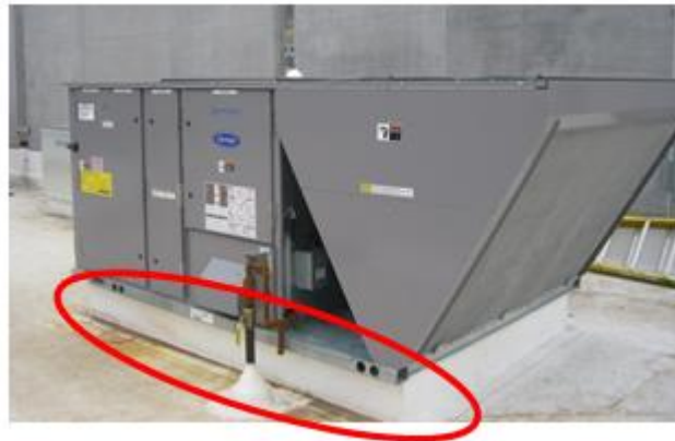
Figure 11- This is a picture taken from the sight showing the lack of any type of vibration control.
