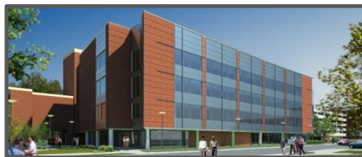
Figure 1: Moore Building Addition
