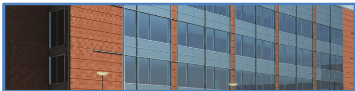
Figure 5: Façade of Moore Building Addition
