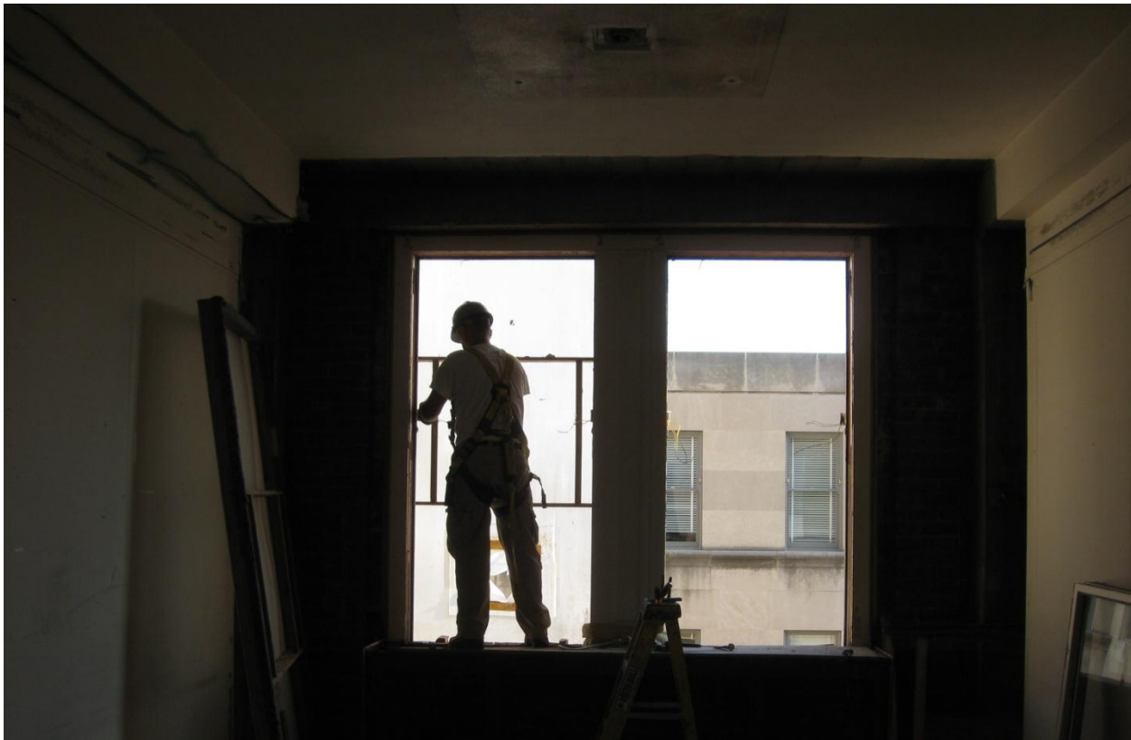
Laborer Working On Window Frame
