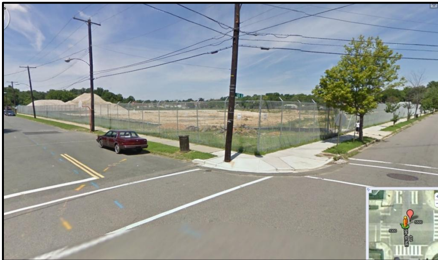
Figure 9: View after Demolition from 55th and EADS Intersection (Courtesy Google Maps)
