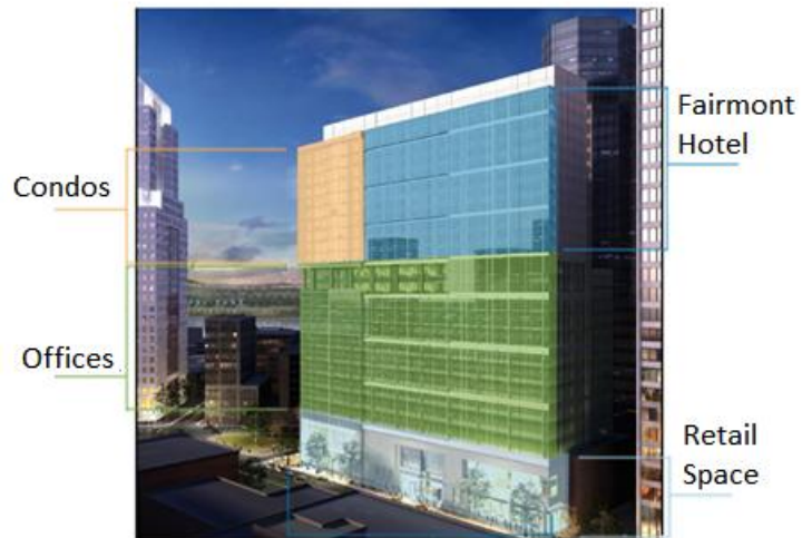
Figure 1- Three PNC Occupancy Layout
