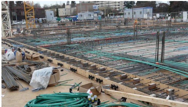
Figure 12 - Post Tensioned System 1
