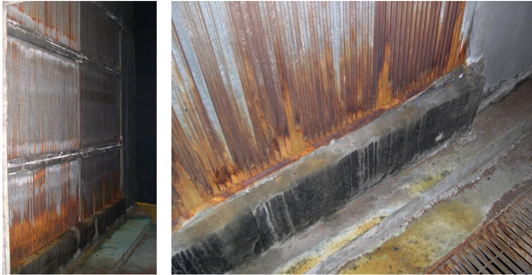
Figure 4-a and b: AHU-S1 and S2 cooling coils, respectively (courtesy of JMT)
