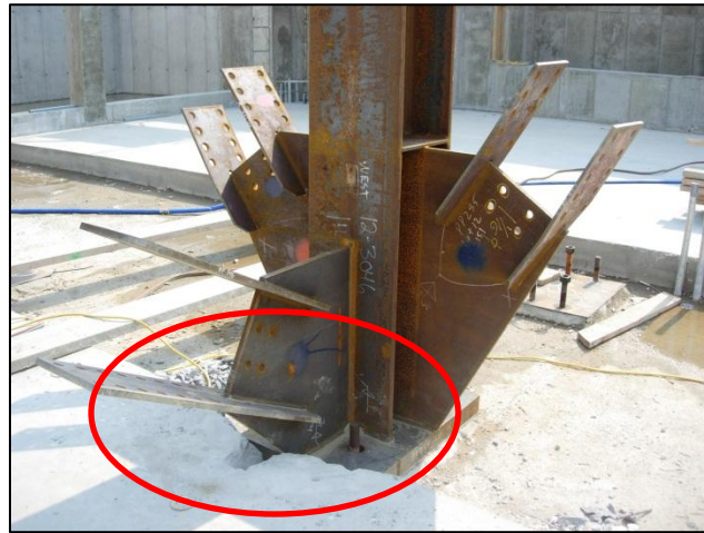
Figure 7: Foundation braced frame connection issues
