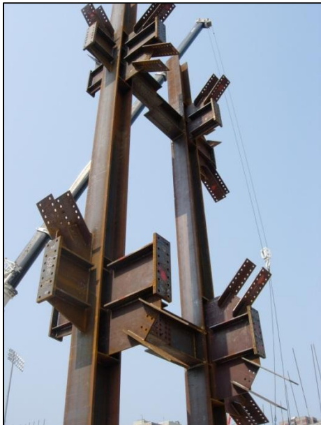
Figure 6: Connection construction photo
