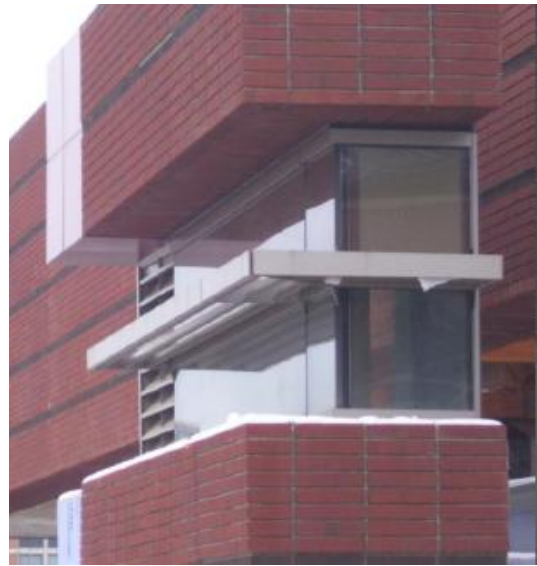
Figure 2: Mockup of building enclosure, including precast panels courtesy of Rvan Solnoskv
