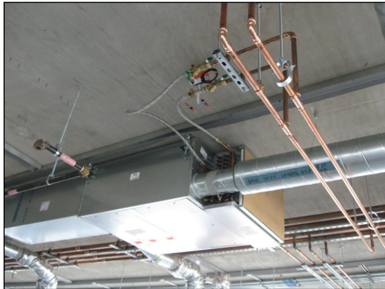
Figure 47- FPIU in Plenum Space
