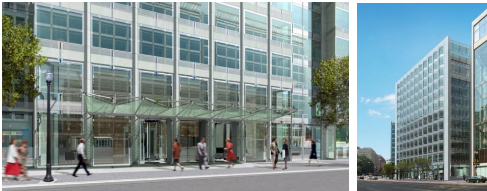
Figure 2 Main Lobby Entrance facing K Street (left) and perspective of curtain wall system (right)
