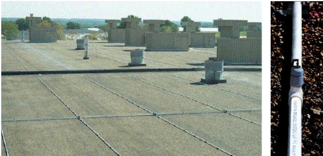
Figure 12 Sprinkool System Installation
