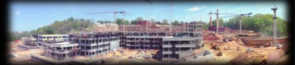
APRIL 2011 PROGRESS PHOTOGRAPH
