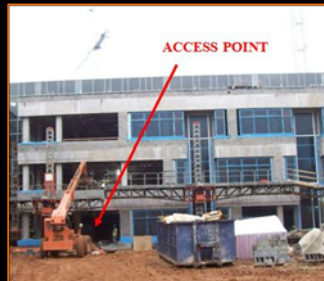
BUILDING ACCESS INTERFERENCE
