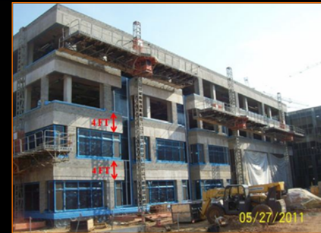
MASONRY CORNER POLE RESTRICTIONS
