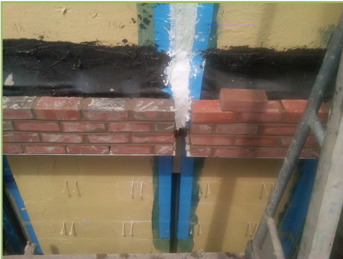
Figure #12 – Expansion Joint Waterproofing
