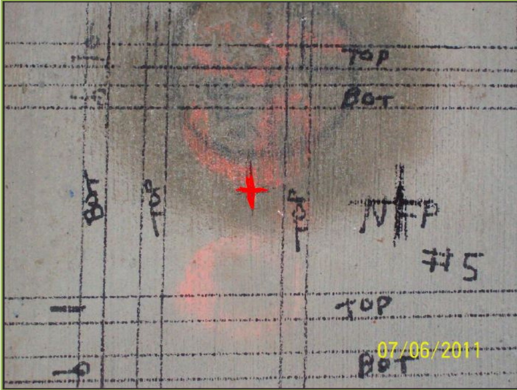
Figure #3 – Core Drilling Location Example – Courtesy of Clark Construction
