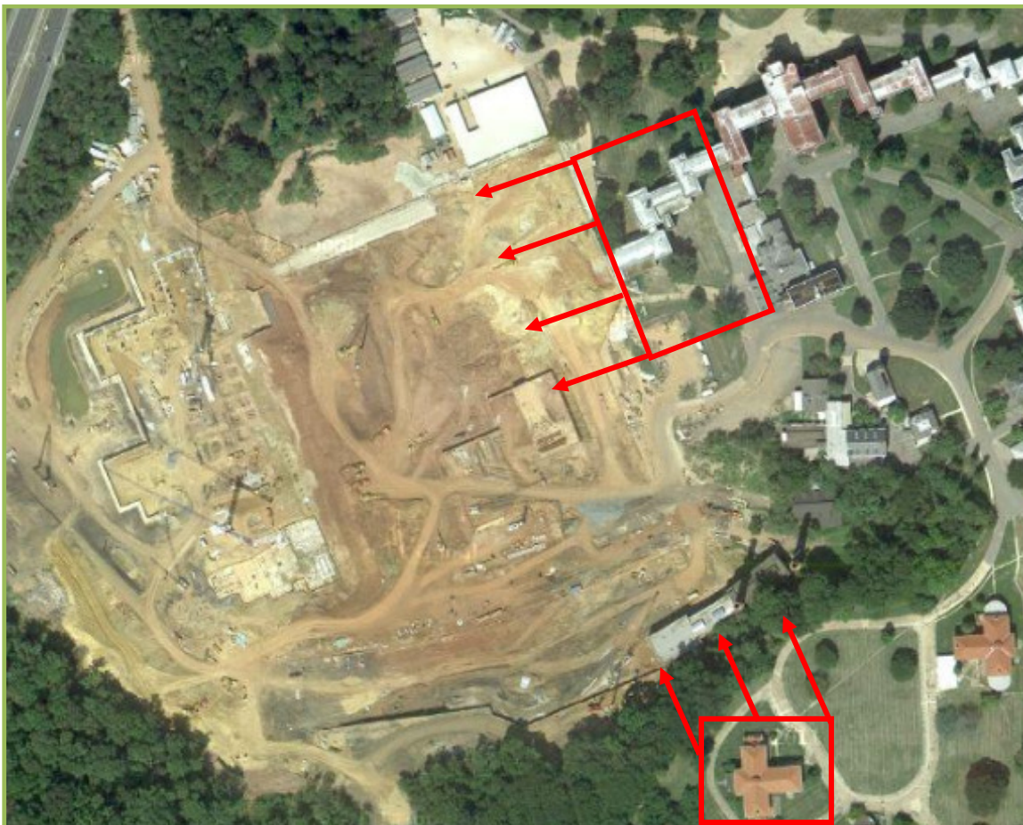
Figure #1 – Existing Structures Affecting the Hillside
