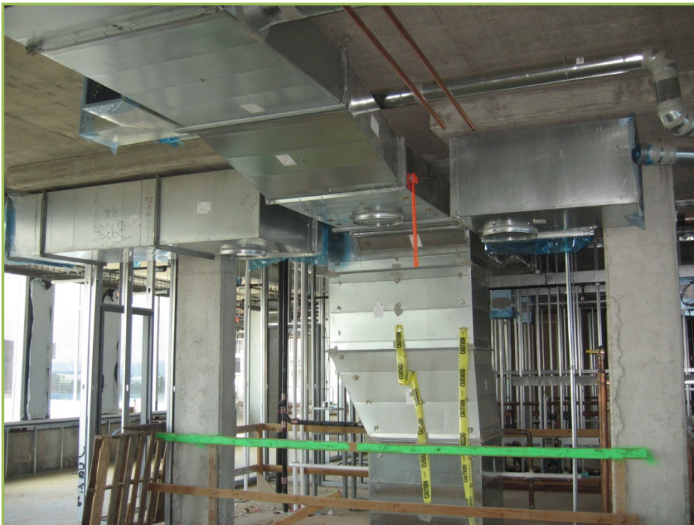
Figure #4 – Unaffected Mechanical Shaft – Courtesy of Clark Construction
