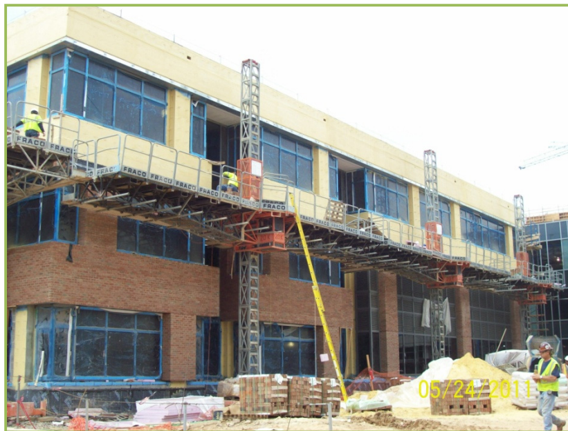
Figure #13 – Recessed Façade Features – Courtesy Clark Construction
