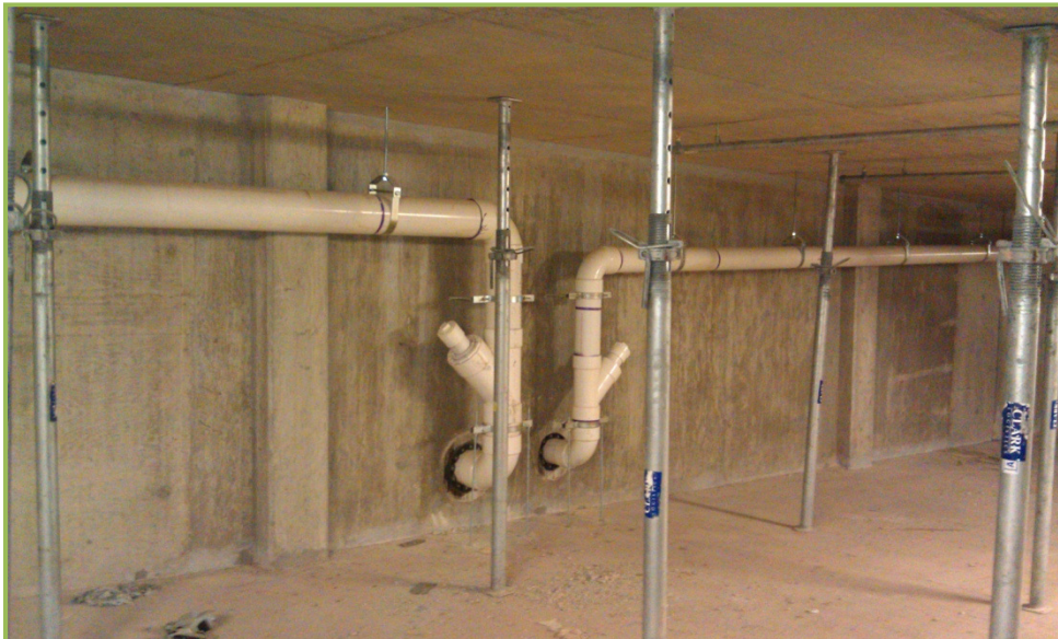
Figure #5 – Unpainted Garage Interior – Courtesy of Clark Construction
