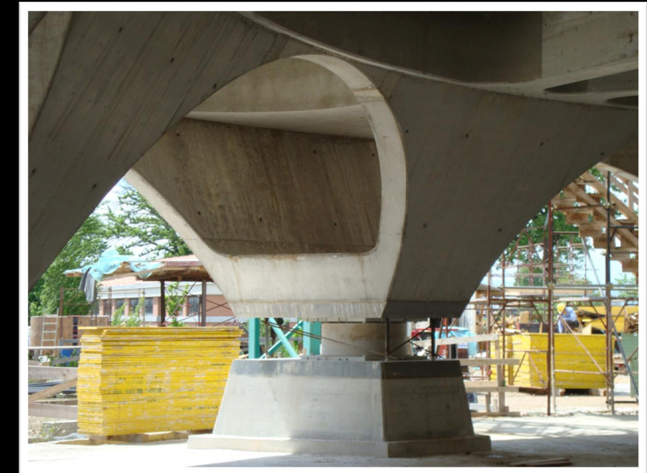
Emergency Management Centre of Foligno, Italy
