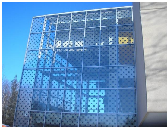
Figure 10- Photovoltaic glazing system of 50% transparency from Atlantis Energy Systems
