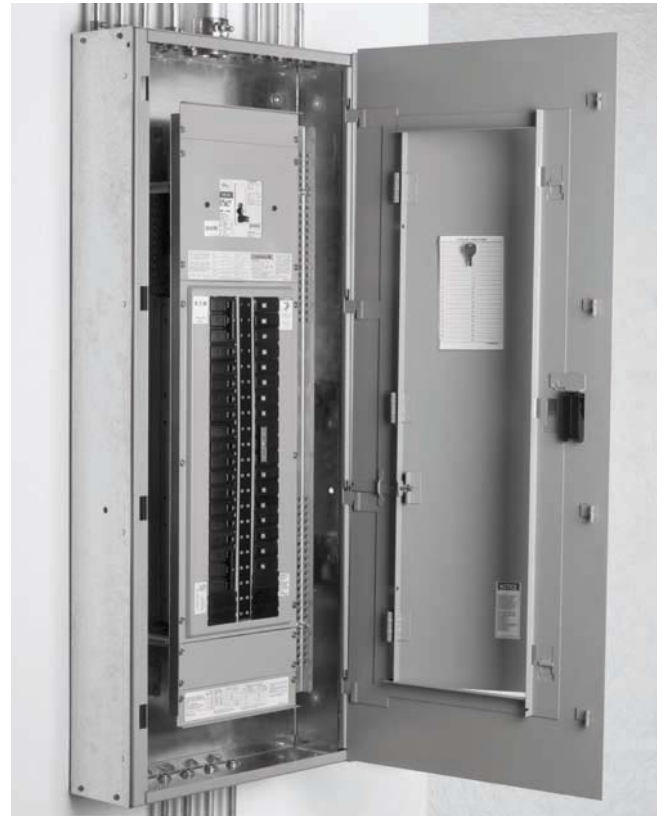
Trim Hanging on Surface Mounted Box
