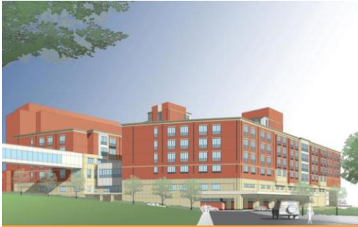
PHASE ONE 6-STORY HOSPITAL
