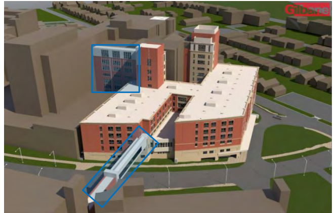
Figure 1 – Pedestrian Bridges Image courtesy of Gilbane Construction
