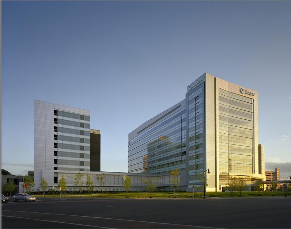
Roberts Pavilion Camden, NJ
