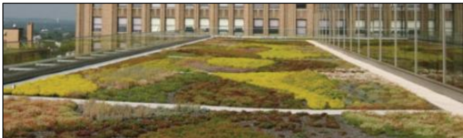
Figure 9: Hydrotech Garden Roof Assembly (American Hydrotech Inc., 2013)
