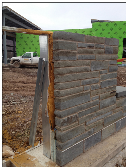
Figure 11; Façade Connections
