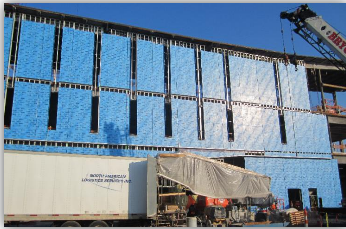
Figure 3: Prefabricated Metal Wall Panels
